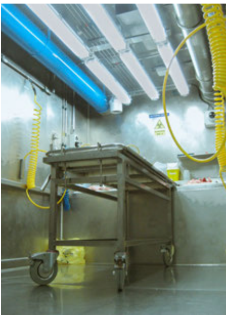
View of the Autopsy suite within the BSL4 container. The yellow hoses carry air to the operators in their BSL4 suits.
